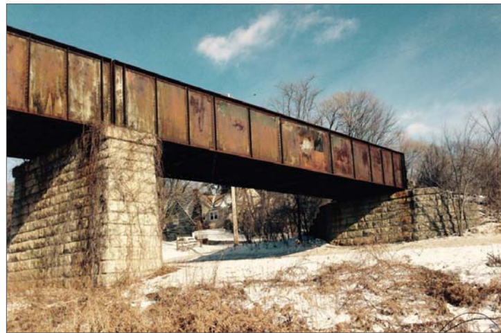
Figure 1. Canadian National Viaduct Over Riverside Drive. Source: GRAEF.
