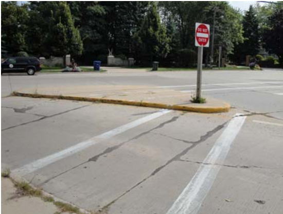
The poor crosswalk continuity, absence of curb cuts, and placement of the sign/signal posts indicate that pedestrian accessibility was not emphasized when these “pork chop” islands were installed.
