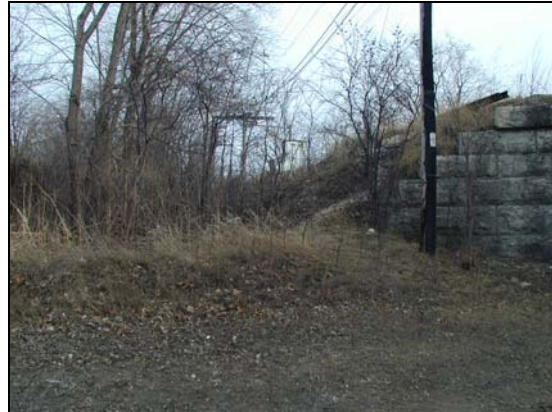
Northeast bank of the railroad trestle
