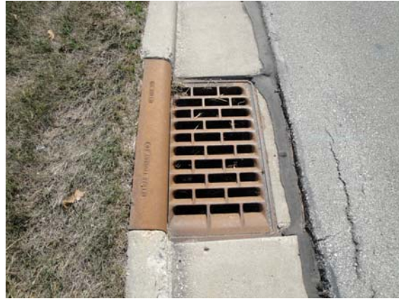
Parallel bar grates can be hazardous to bicyclists... ..but perpendicular grates allow bikers to cross them safely.
