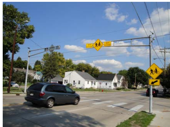
...but flashing overhead pedestrian crossing signals could be easily seen by approaching drivers.
