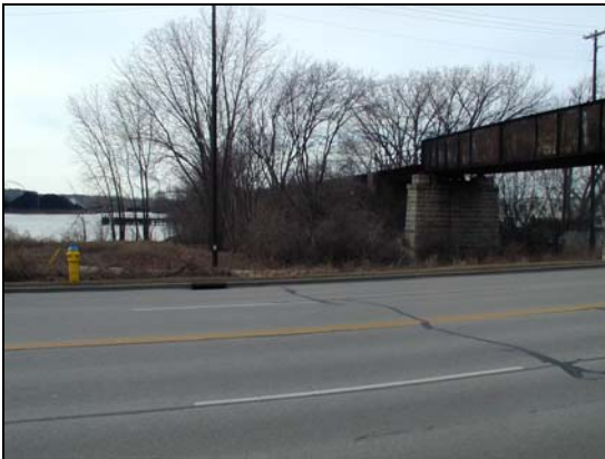
Southwest bank of the railroad trestle
