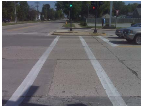
The poor crosswalk continuity, absence of curb cuts, and placement of the sign/signal posts indicate that pedestrian accessibility was not emphasized when these “pork chop” islands were installed.
