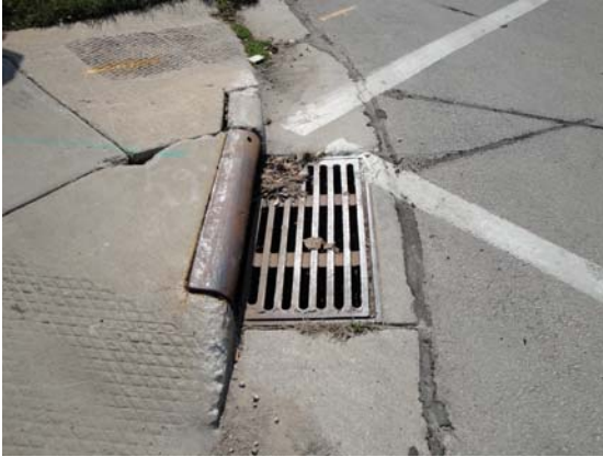
Parallel bar grates can be hazardous to bicyclists... ..but perpendicular grates allow bikers to cross them safely.
