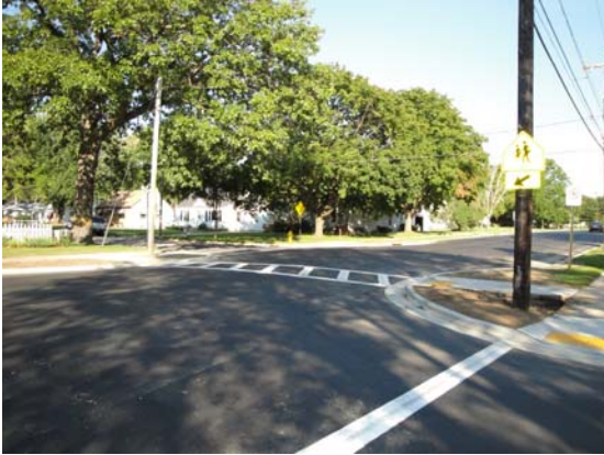
Curb extension near Dickinson Elementary School in De Pere.
